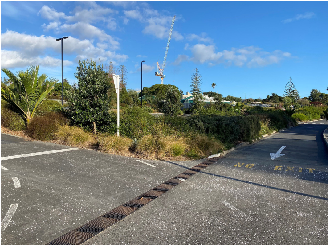
Fig. 6 In 2023, 13 years after construction (shown in Fig. 4), the plantings of the vegetated swale at ABG are well established and the swale channel can no longer be seen. Photo: Emma Simpkins.
