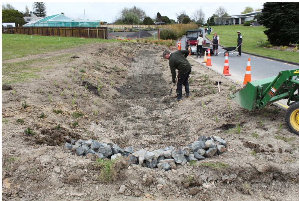
Fig. 4 Construction of the vegetated swale in 2010 at ABG. Photo: ABG.
